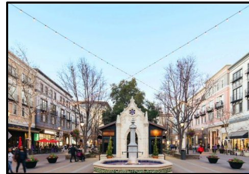
Santana Row, San Jose Retail / Office / Residential
